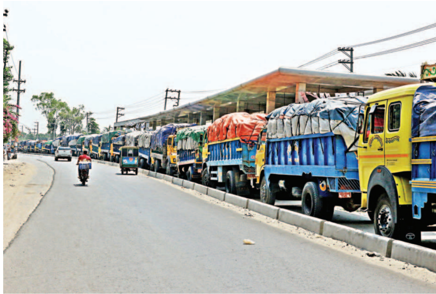
Trucks are parked illegally in front of an under-construction Bus Rapid Transit station near Gazipur jail, hampering the construction work. The vehicles were waiting there yesterday to offload goods at nearby factories.
