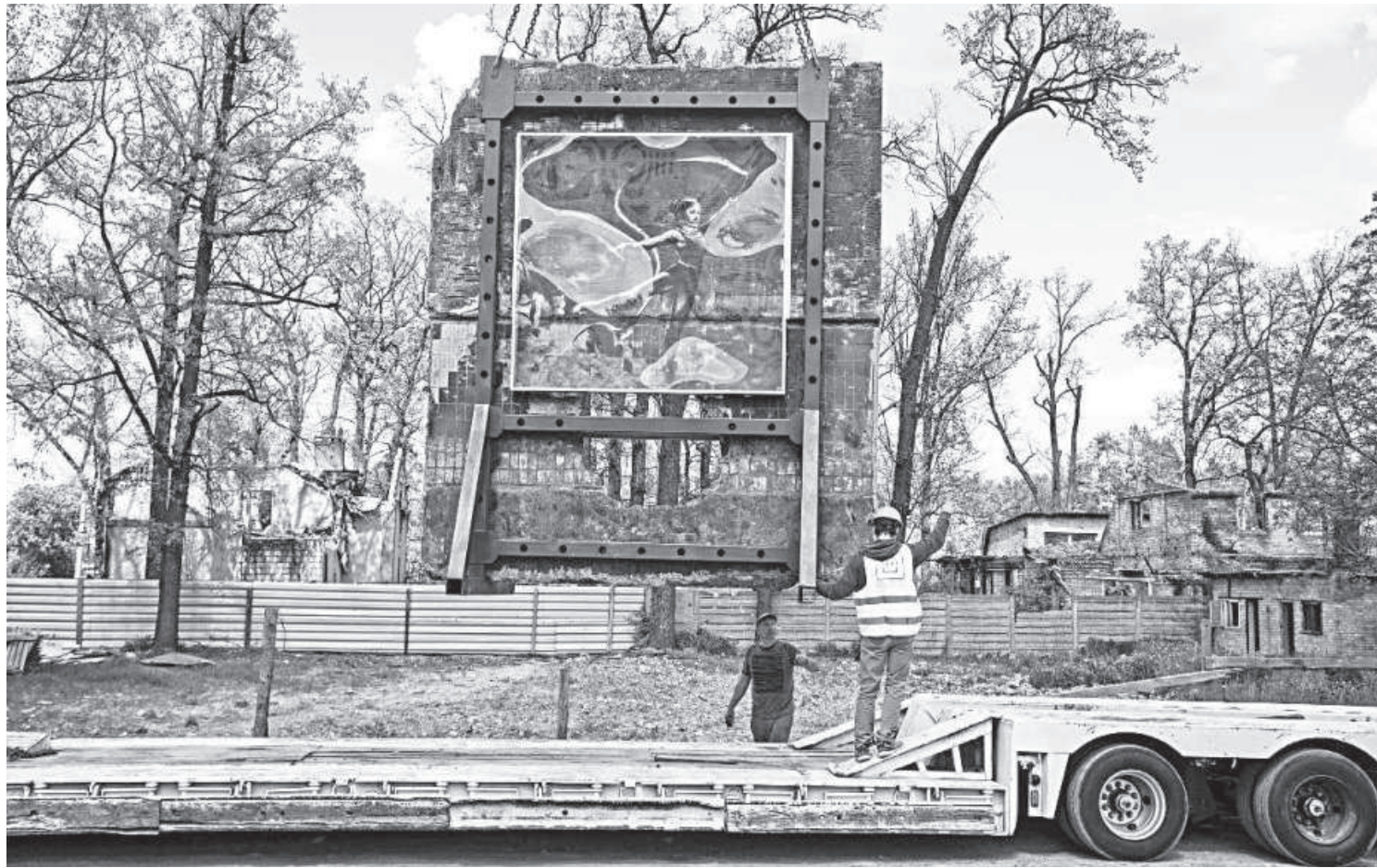
Workers unload from a semi-truck a part of a wall with the work of world-renowned graffiti artist Banksy which was dismantled from a residential building heavily damaged during Russia's attack in the town of Irpin, outside of Kyiv, Ukraine yesterday.
