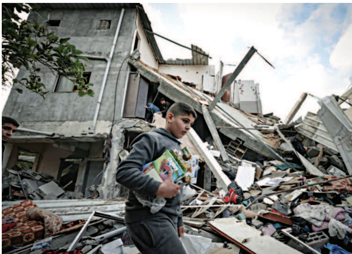
A Palestinian child carries belongings salvaged from the rubble of a building, damaged in Israeli air strikes on Gaza city yesterday. PHOTO: AFP
