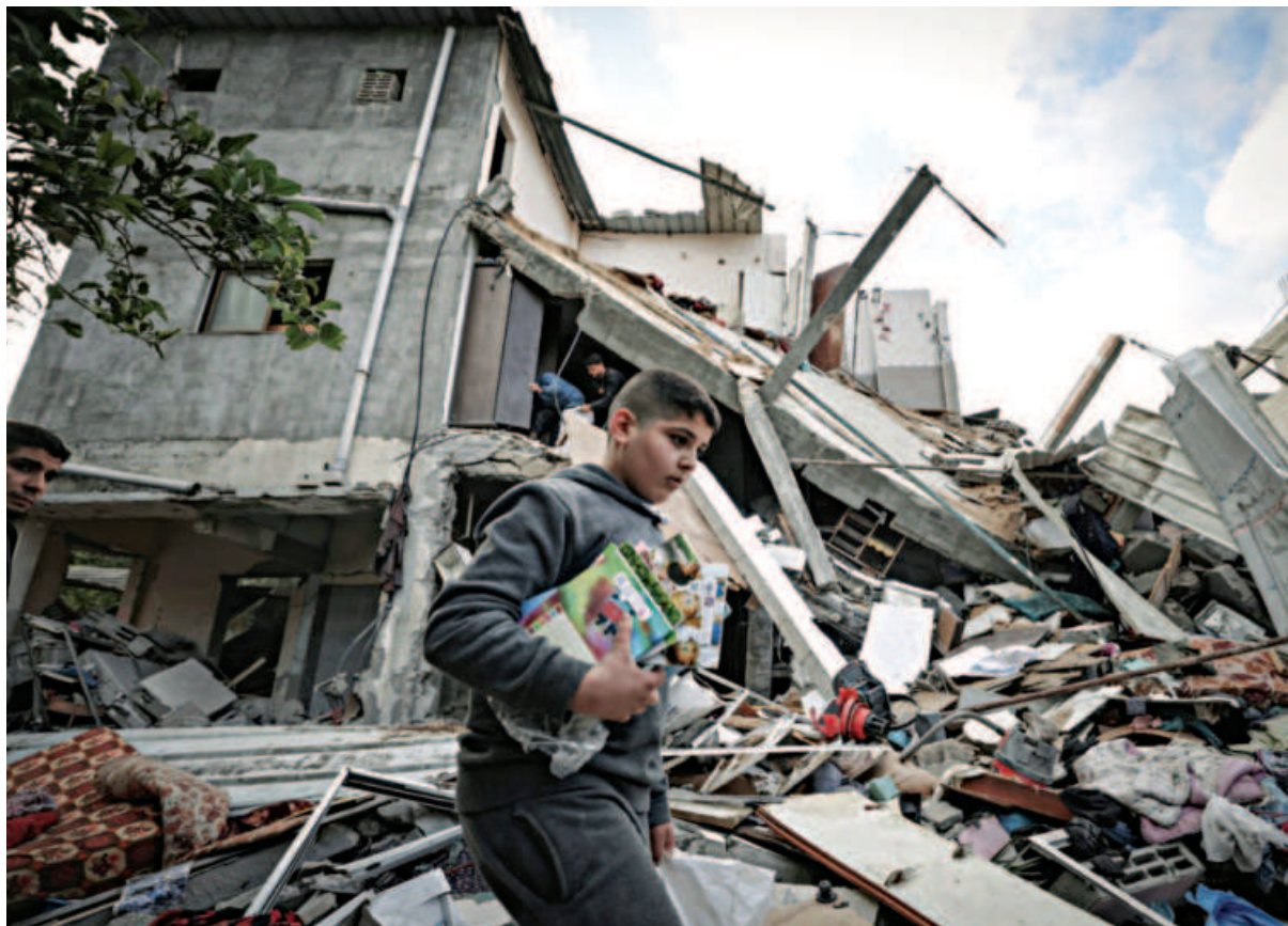
A Palestinian child carries belongings salvaged from the rubble of a building, damaged in Israeli air strikes on Gaza city yesterday. PHOTO: AFP
