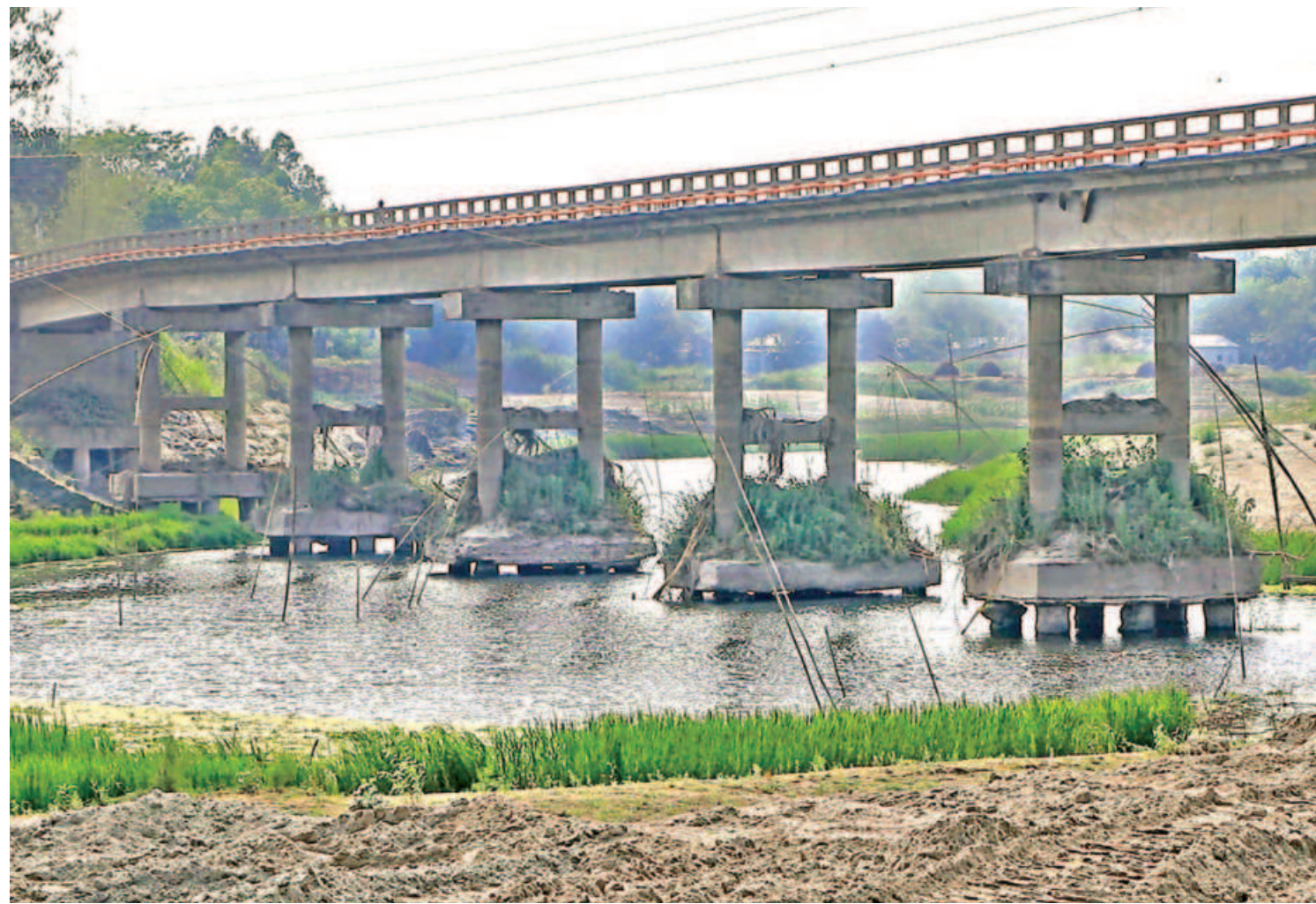
Illegal sand lifting from the Dhaleswari river at Charabari in Tangail Sadar upazila threatens a nearby bridge. People of five unions use this bridge to get to the district town. The photo was taken recently.
