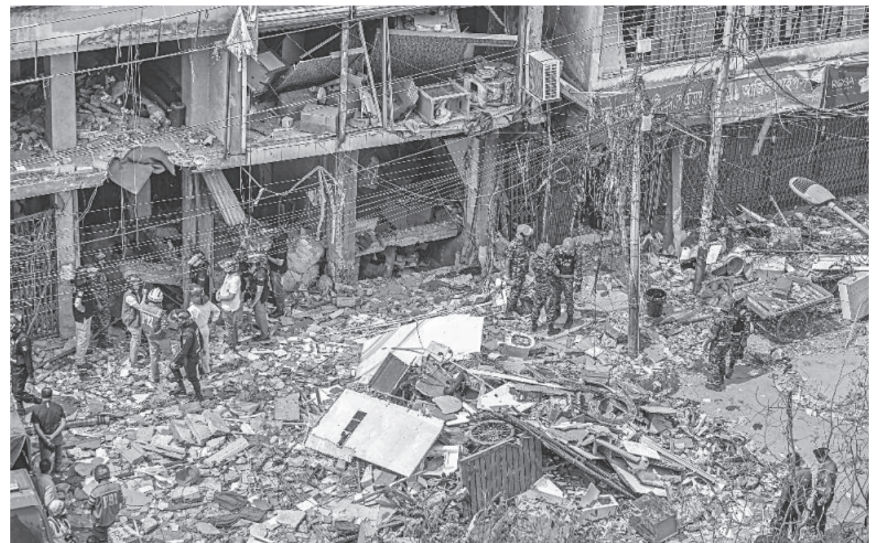
The horrific explosion in Gulistan, Dhaka on March 7, 2023, which killed 22 people, happened because of accumulated gas and could've been easily prevented.
