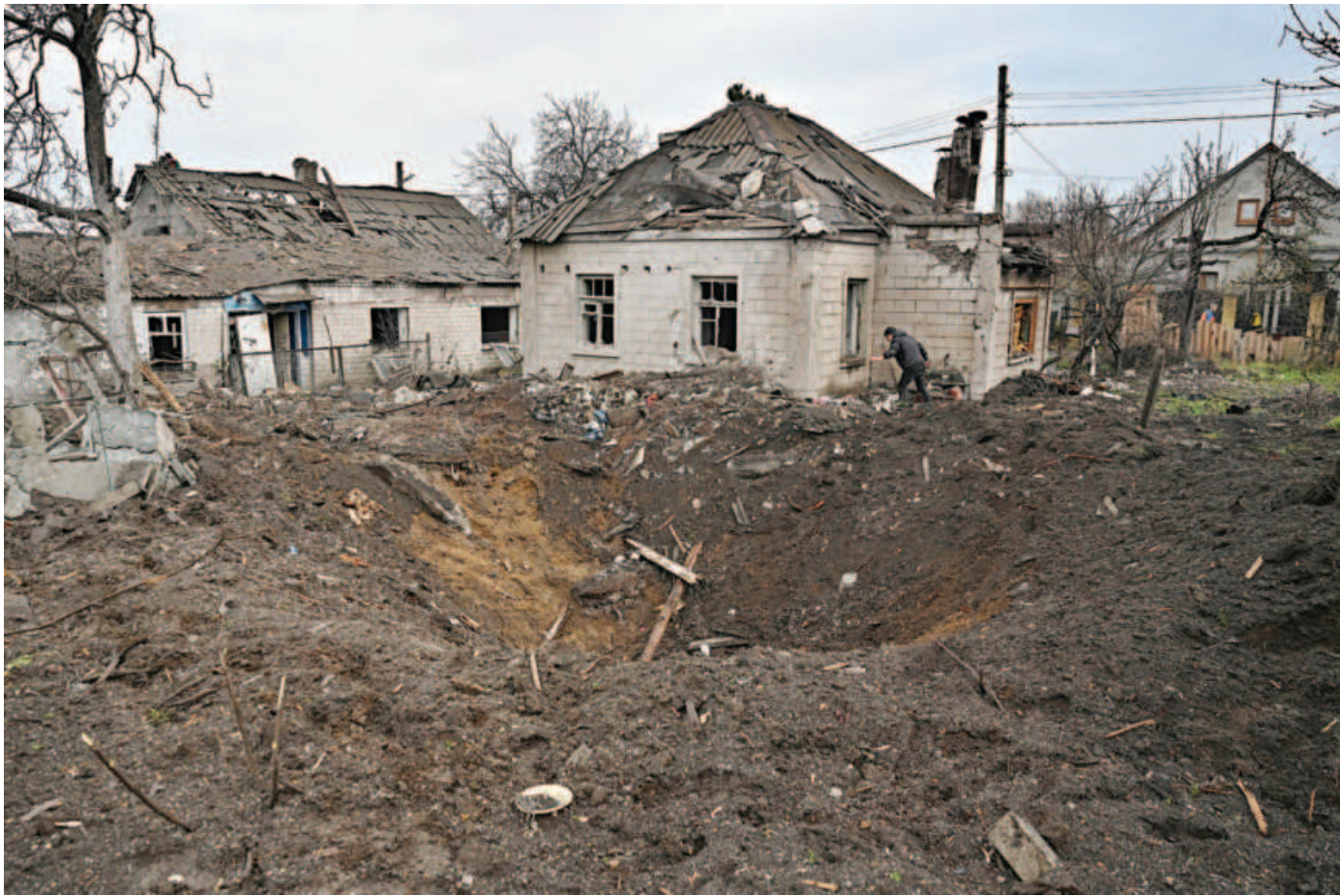
A local resident removes debris from his house damaged by a Russian missile strike, amid Russia's attack on Ukraine, in Zaporizhzhia, Ukraine yesterday.
