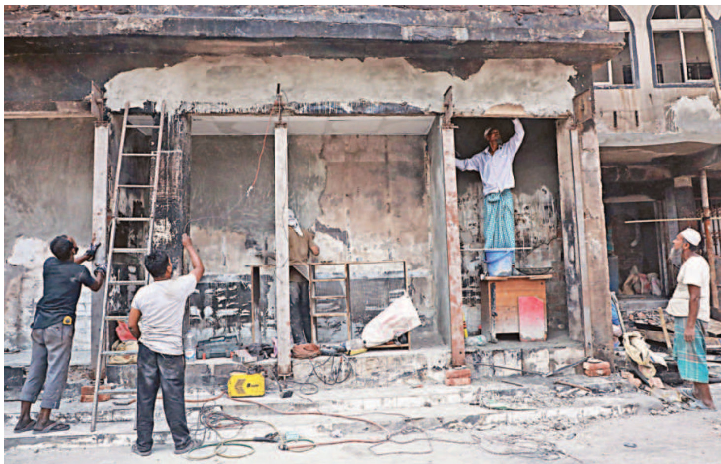
Like other nearby establishments, these shops opposite to Bangabazar shopping complex in Dhaka's Gulistan area were damaged during a recent fire that broke out at the popular apparel retail hub. Here, workers are seen conducting repairs in hopes of reopening the store before Eid-ul-Fitr. The picture was taken yesterday.
