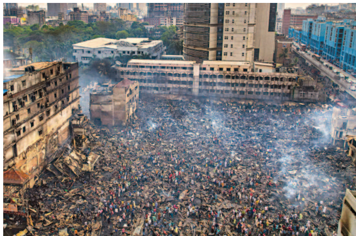
Bangabazar Shopping Complex was still smouldering yesterday after a devastating fire gutted it on Tuesday. Many shop owners said they may slide into poverty after losing their investments.
