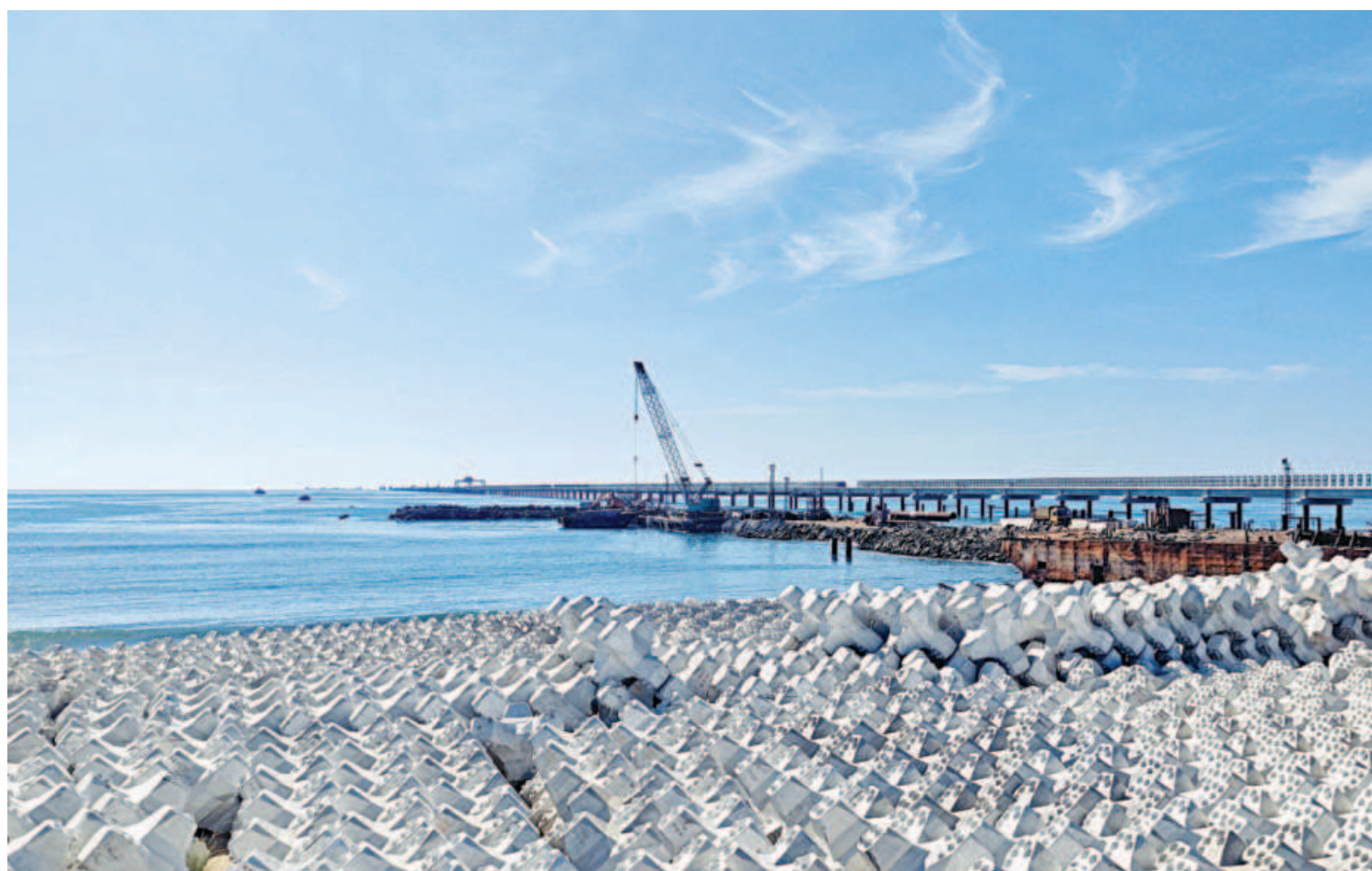
A view of an under-construction coal jetty of a power plant on the coastline near India's southern tip in Udangudi of Tamil Nadu. Intense summer heatwaves, a colder-than-usual winter in northern India and an economic recovery led to a jump in electricity demand, forcing India to crank up output from coal plants and solar farms as it scrambled to avoid power cuts.
