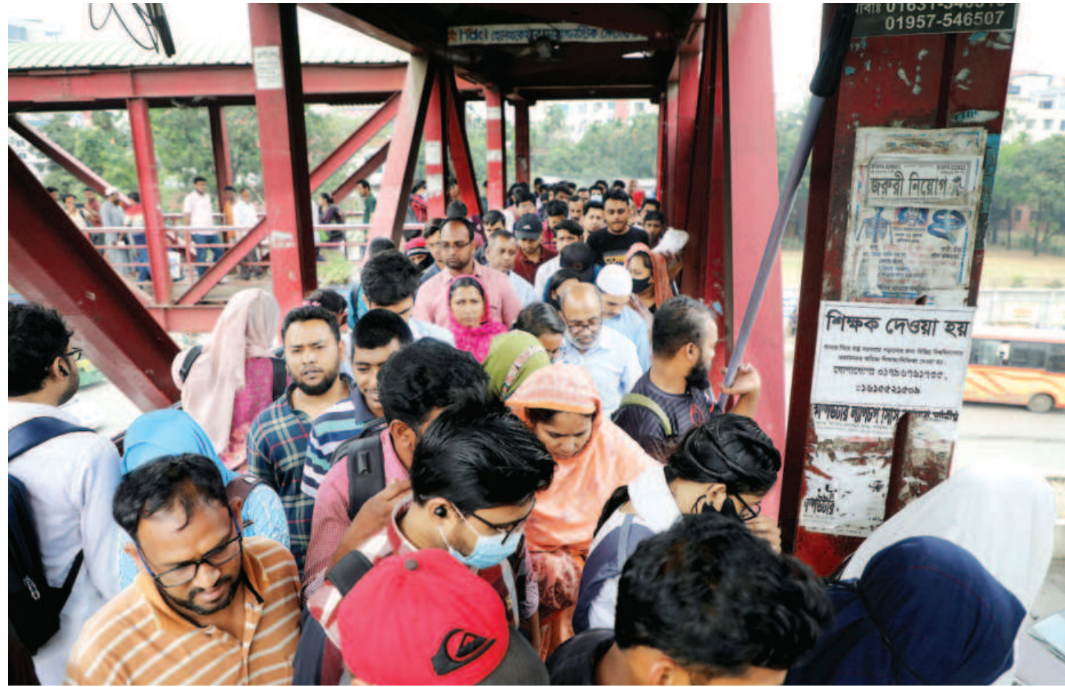
Pedestrians struggling to cross a footbridge at the Shishumela intersection in the capital's Shyamoli area. As the footbridge itself and the stairways leading up to it are both very narrow, it becomes rather chaotic when a lot of people, many of whom are patients of nearby hospitals, cross together. The photo was taken recently.
