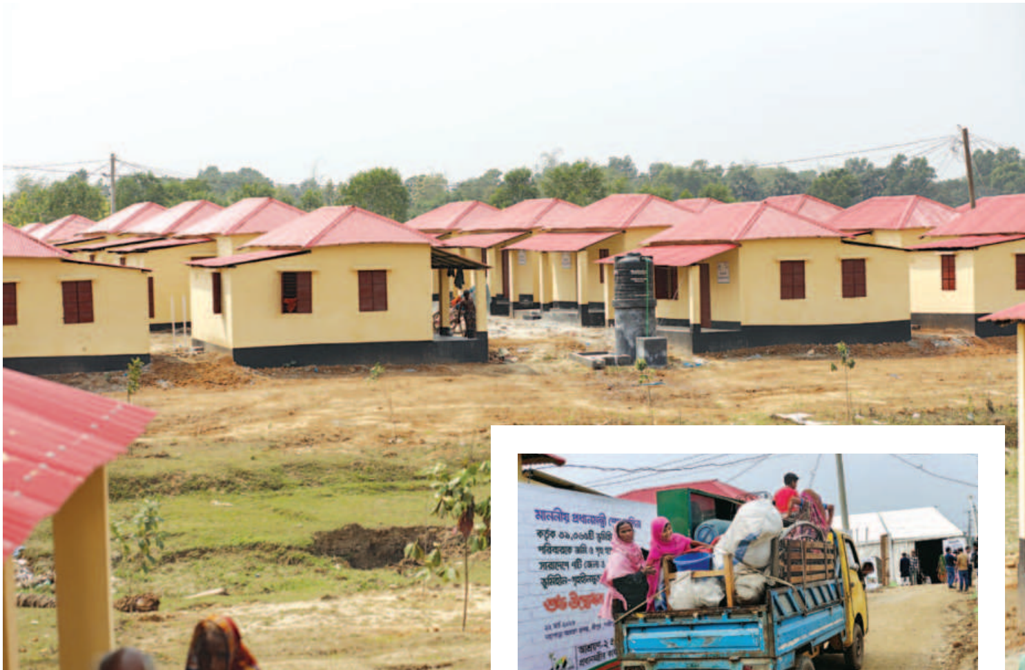
A portion of the Ashrayan-2 housing project site in Gazipur's Nayapara. Inset, one of the 142 families moving into the new home on Wednesday.
