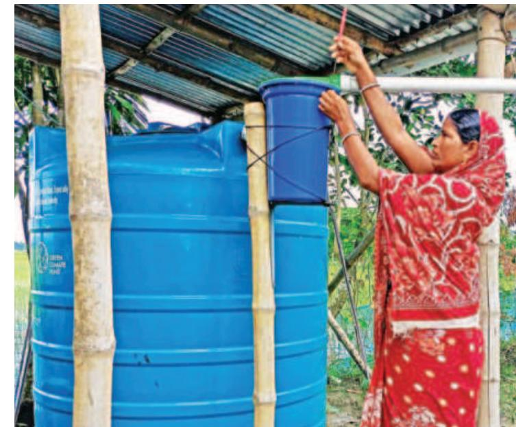
"We installed a 60 square feet tin roof as a self-catchment system to collect rainwater in every house. The water passes through a primary filtration system to remove larger particles, followed by a pre-filtration unit to remove solid substances and
