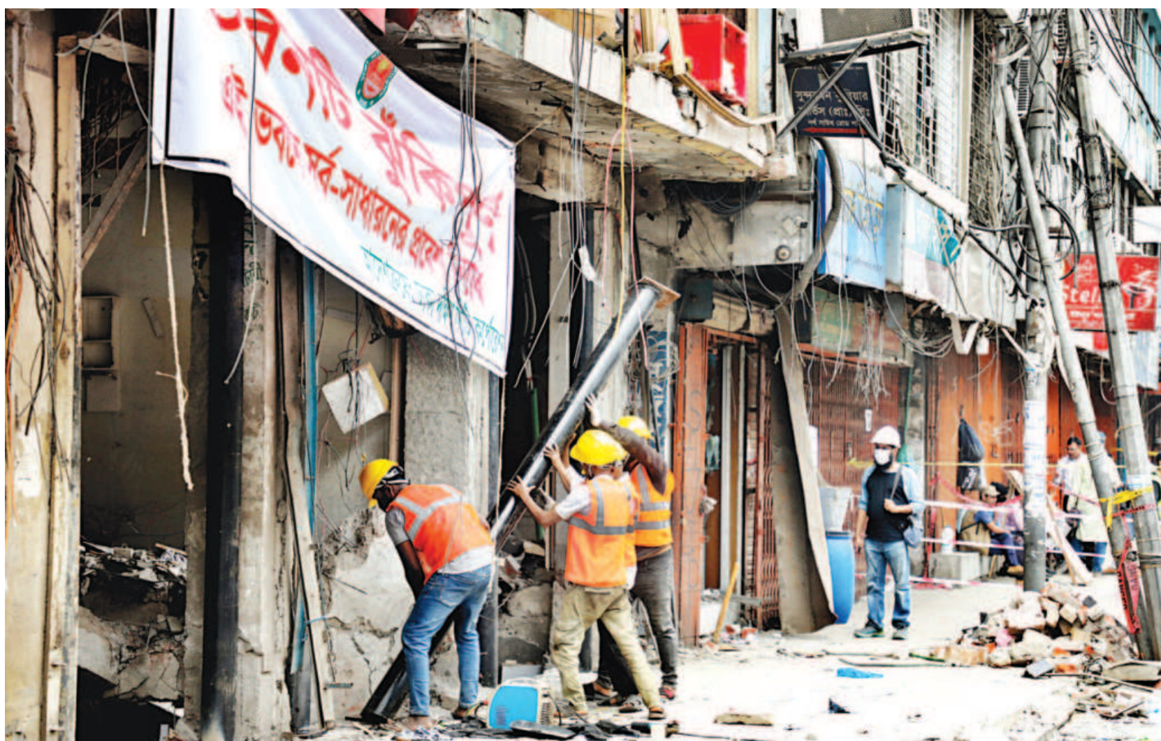
Workers moving an iron pole to prop up a beam of the seven-storey building on North South Road in the capital's Siddikbazar yesterday. A massive blast at the building on Tuesday killed at least 22 people and injured over 100 others.
