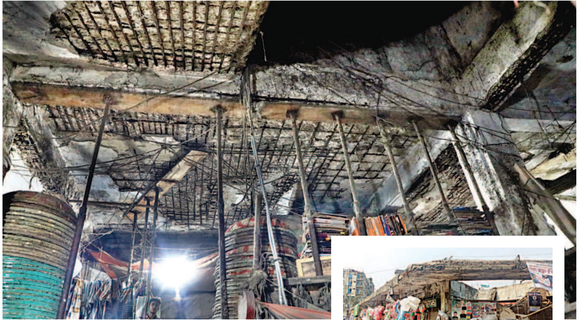
Only the bare rods remain as the plasters have fallen off at a building of Karwan Bazar kitchen market in the capital. Four such buildings in the area are labelled by the city corporation as risky, but tens of thousands of people buy and sell goods at these buildings every day. Inset, Rayerbazar kitchen market is also in a sorry state.
