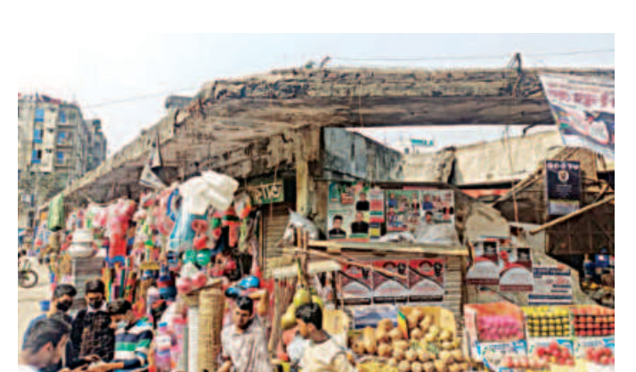
Only the bare rods remain as the plasters have fallen off at a building of Karwan Bazar kitchen market in the capital. Four such buildings in the area are labelled by the city corporation as risky, but tens of thousands of people buy and sell goods at these buildings every day. Inset, Rayerbazar kitchen market is also in a sorry state.
