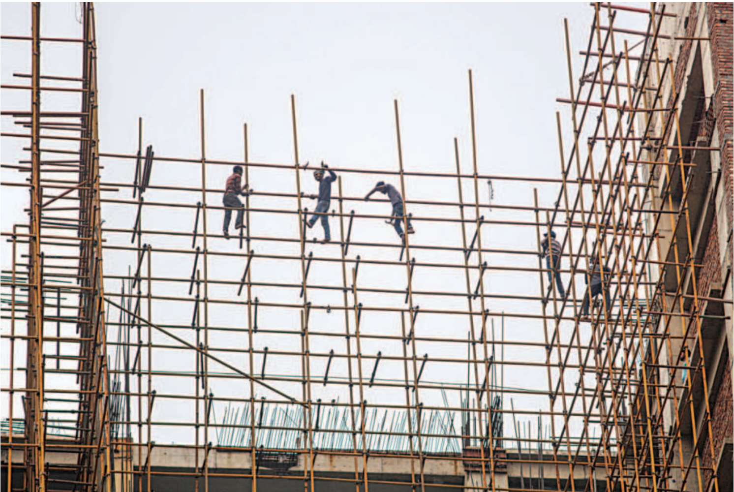
Workers building a scaffolding at the construction site of a highrise of Sarkari Karmachari Hospital in the capital’s Fulbaria. They appear to be not tethered to anything and a slip could be fatal. The photo was taken yesterday.
