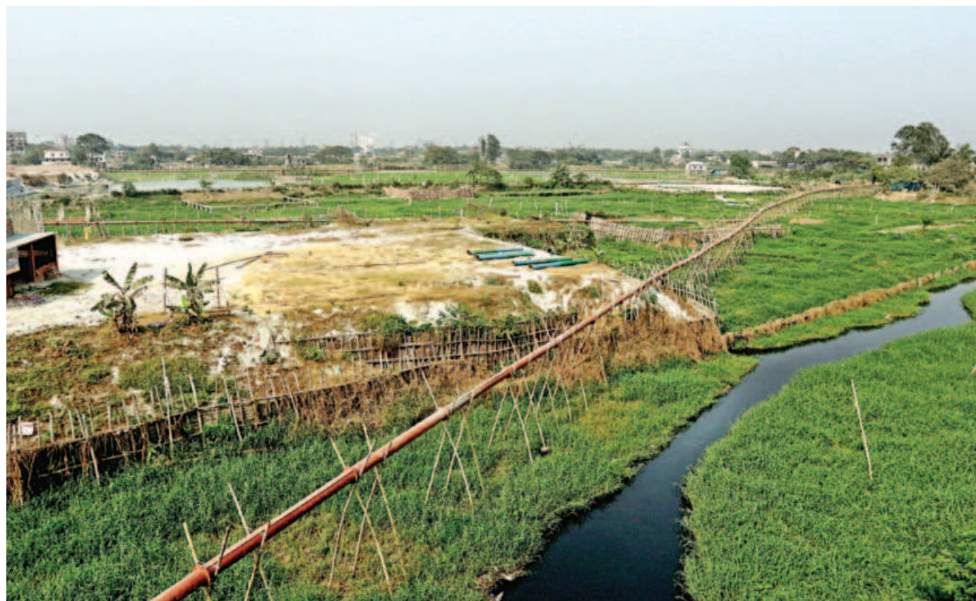
Sand-filling in a wetland, also considered a flood zone, goes on unabated in Khilgaon's Nagdarpar area in the capital. Land grabbers have put up signs on water bodies and built structures there to develop housing settlements. Experts have warned that filling up marshlands would make the capital highly vulnerable to earthquake hazards and other natural disasters, while Prime Minister Sheikh Hasina on numerous occasions urged that lowlands and flood zones be kept safe. However, her request seems to have fallen on deaf ears. The photo was taken yesterday.
