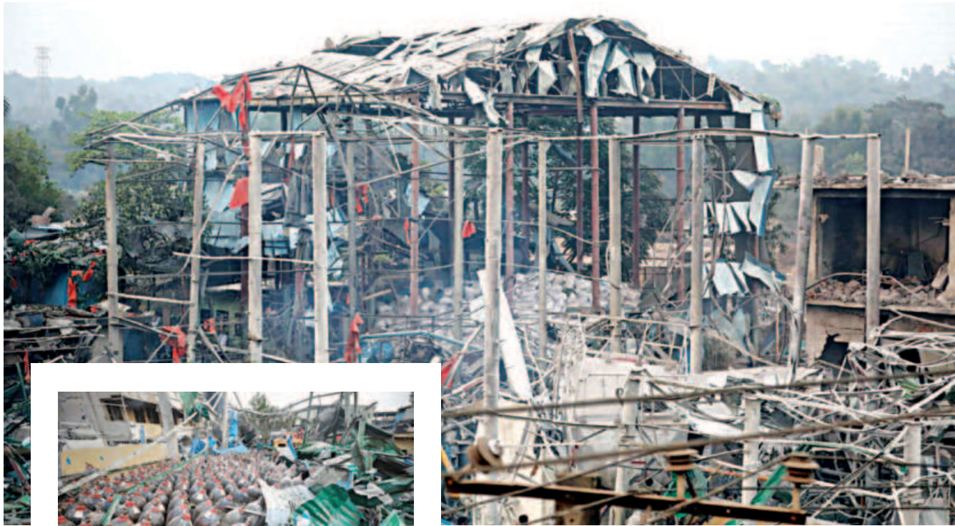
The remains of Seema oxygen plant in Sitakunda next to the Dhaka-Chattogram highway after an explosion. The blast sent shards of metal hurtling across hundreds of metres. Inset , oxygen cylinders kept at the plant.
