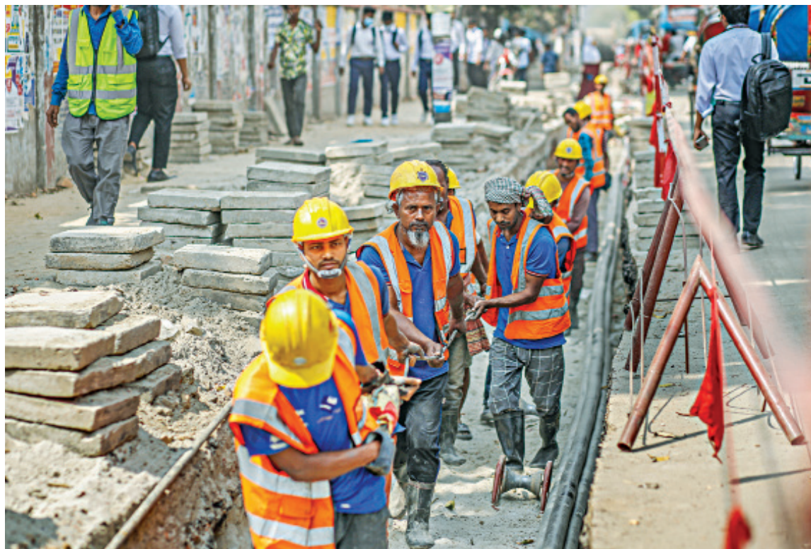
Workers installing underground cables on Satmasjid Road in Lalmatia yesterday. Dhaka Power Distribution Company (DPDC) is conducting the work.
