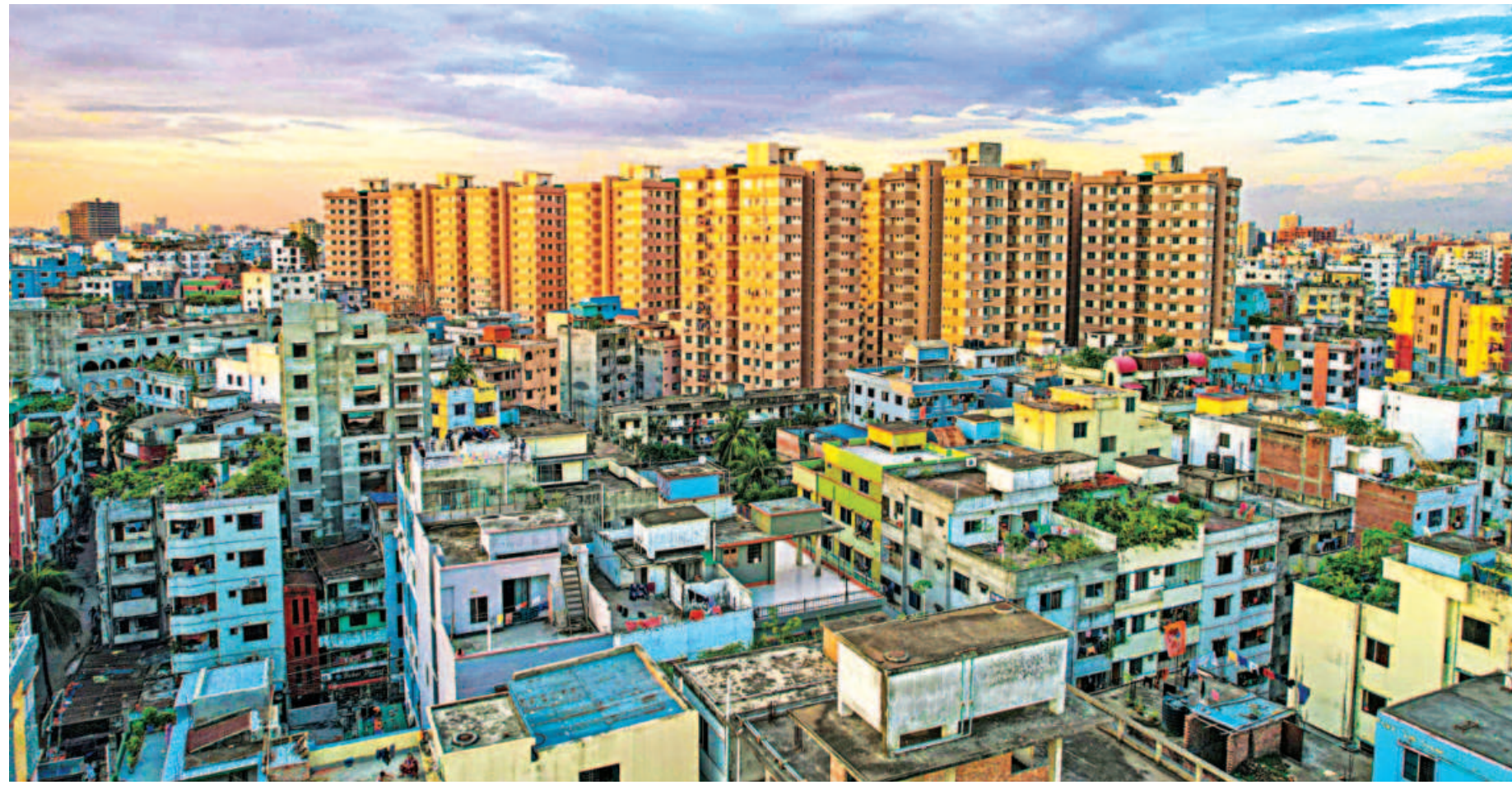
The number of multi-storey buildings is on the rise to meet the housing demand in Dhaka, one of the most populous cities in the world. However, the properties are increasingly going out of the reach of most of its inhabitants owing to skyrocketing prices.
