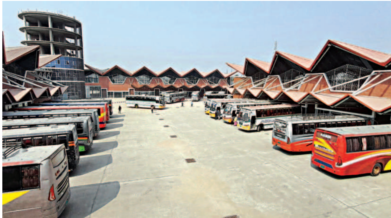
Buses parked at the newly built Kadamtali bus terminal in Sylhet city. The terminal, built on around 8.5 acres by Sylhet City Corporation for about Tk 67 crore, was opened on trial last week. The structure is expected to be formally inaugurated soon. The photo was taken yesterday. PHOTO: SHEIKH NASIR
