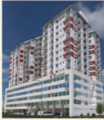
ONGOING Commercial cum Residential Complex SIZE: (252-2093) sft.
