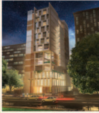
ONGOING Commercial Complex SIZE: (250-2577) sft.
