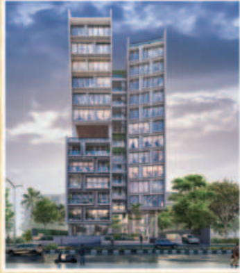
ONGOING Commercial Complex SIZE: (2248-3339) sft.
