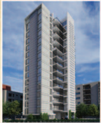
ONGOING Commercial Complex SIZE: (2248-3339) sft.
