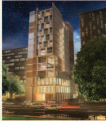
ONGOING Commercial Complex SIZE: (250-2577) sft.
