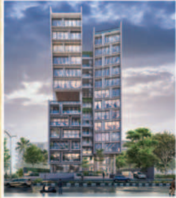
ONGOING Commercial Complex SIZE: (2248-3339) sft.
