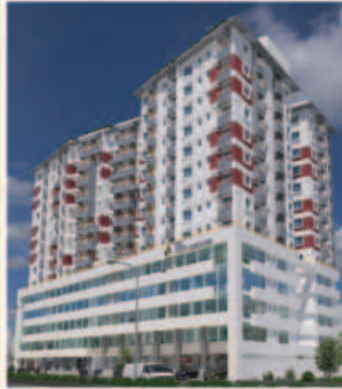
ONGOING Commercial cum Residential Complex SIZE: (252-2093) sft.
