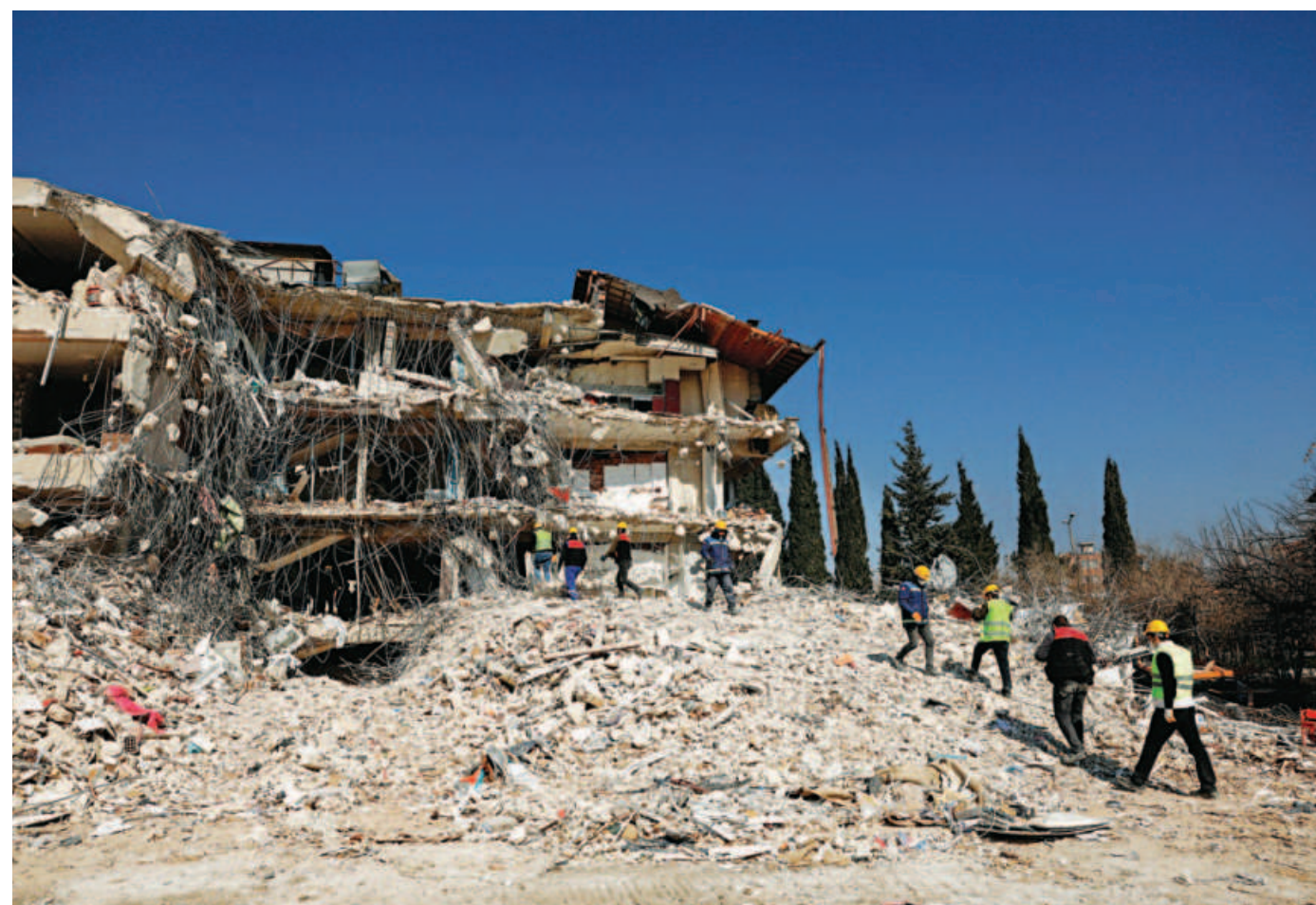
Rescuers work to extract the bodies of a father and a son from under the rubble in the aftermath of a deadly earthquake in Hatay, Turkey yesterday.
