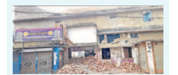
Current state of Malanch Cinema Hall.
