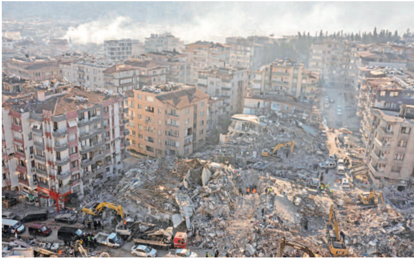
An aerial view shows damaged and collapsed buildings, in the aftermath of a deadly earthquake in Hatay, Turkey, yesterday.
