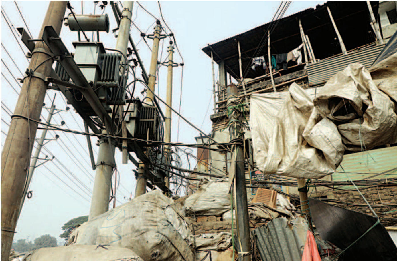
Traders have stacked large bags full of discarded plastic bottles right under electricity transformers at Islambagh in the capital's Lalbagh, putting the area at risk of fire. Some of the bags are in direct contact with electricity cables connected to the transformers. The photo was taken recently.
