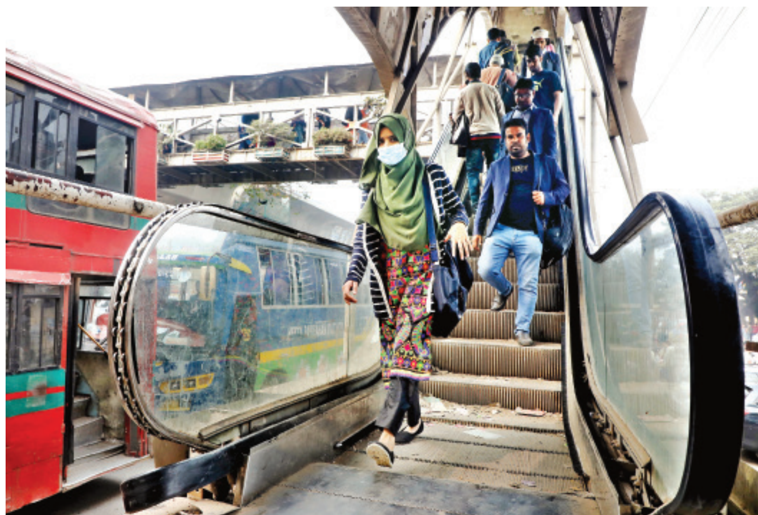
The escalator-equipped footbridge in front of the Dhaka airport used to be a relief for pedestrians, especially the elderly and the ones carrying heavy bags. However, the escalator broke almost two months ago and people now climb up and down the staircase.
