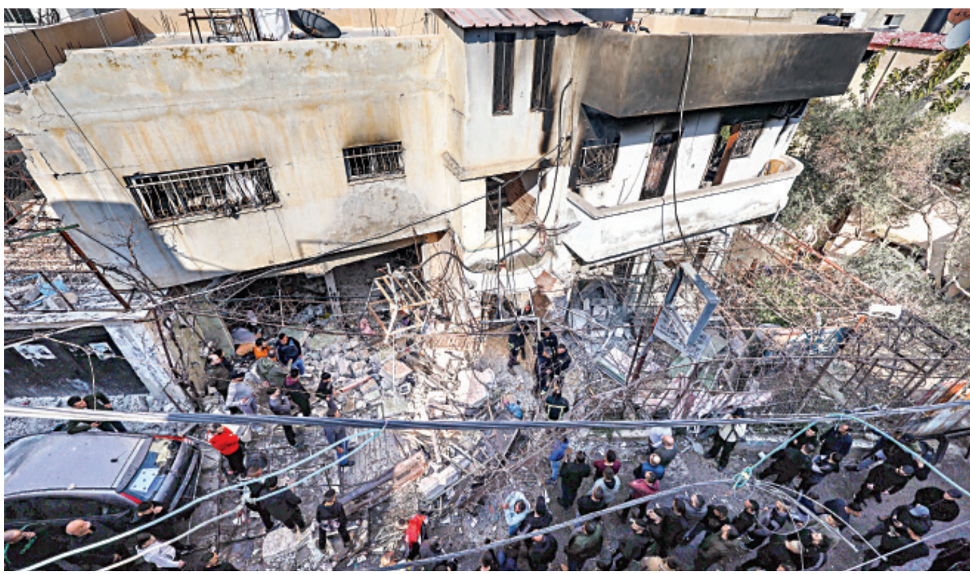
People gather around a building damaged and burned by Israeli troops during a raid on the West Bank's Jenin refugee camp, yesterday. The raid killed 9 Palestinians including an elderly woman, Palestinian officials said, also accusing the army of using tear gas inside a hospital.
