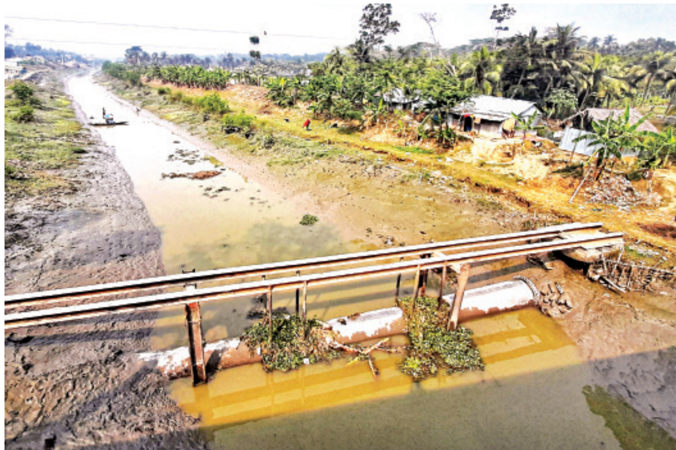
A pipe, installed by Khulna Wasa across the Bhairab river to carry water from the Madhumati to a water treatment plant in Khulna, is obstructing the flow of the river and movement of boats in Mulghar area of Bagerhat's Fakirhat upazila. Bangladesh Water Development Board had excavated the Bhairab three years ago, but the soil, kept on the banks, slid into the river again during the rainy season, causing a loss of navigability. The photo was taken on Sunday.
