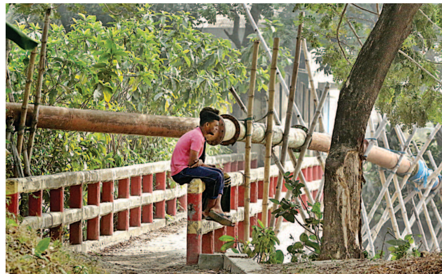
A metal pipe set up over the walkway along the Buriganga, hindering movement of pedestrians. Traders use engines to illegally unload sand from vessels and pump it to the shore through this pipe. The authorities seem to have turned a blind eye. The photo was taken from Aliganj in Narayanganj's Pagla area recently.
