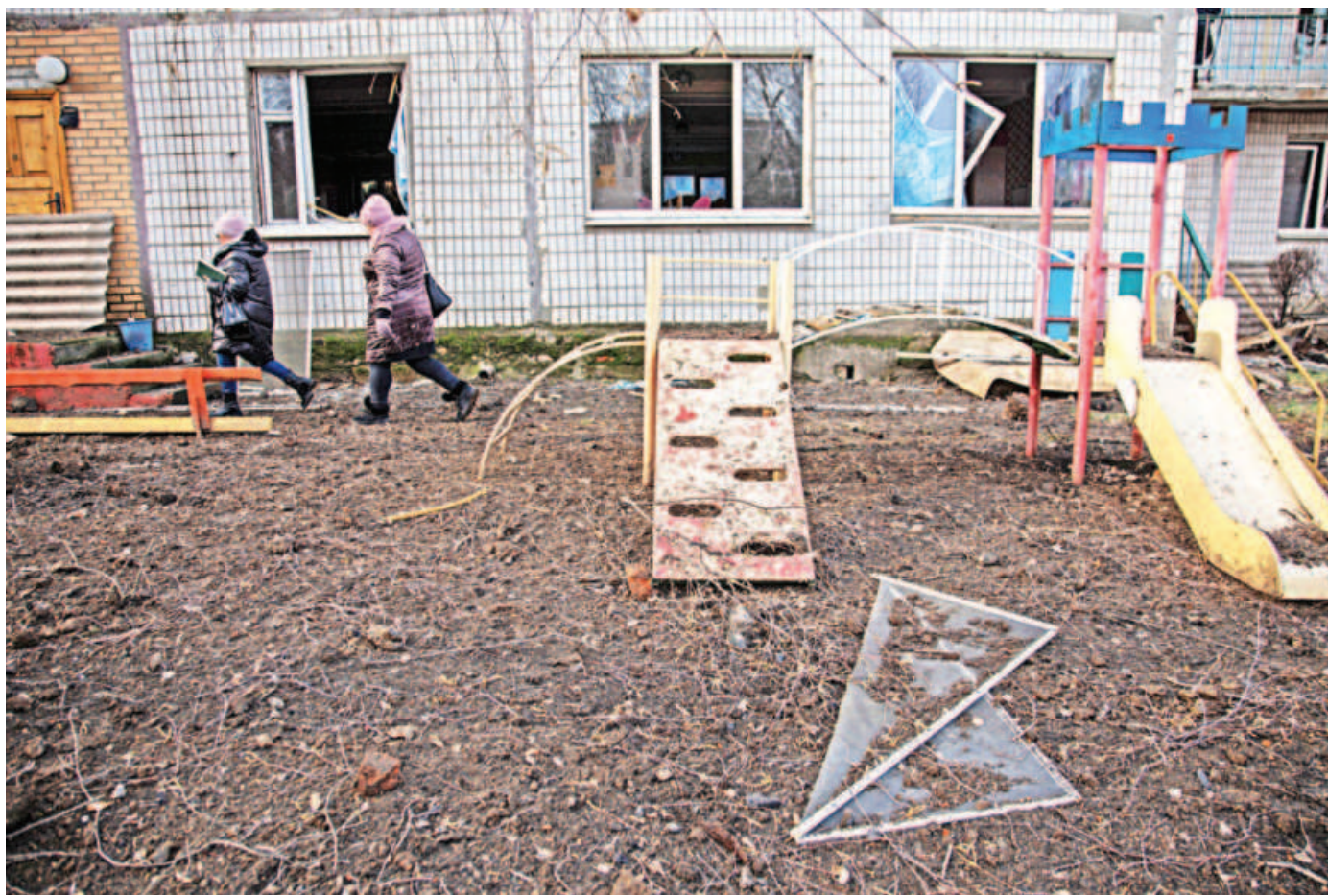
Women walk next to a kindergarten building damaged by a Russian missile strike, amid Russia's attack on Ukraine, in Kramatorsk, Donetsk region, Ukraine yesterday. PHOTO: REUTERS
