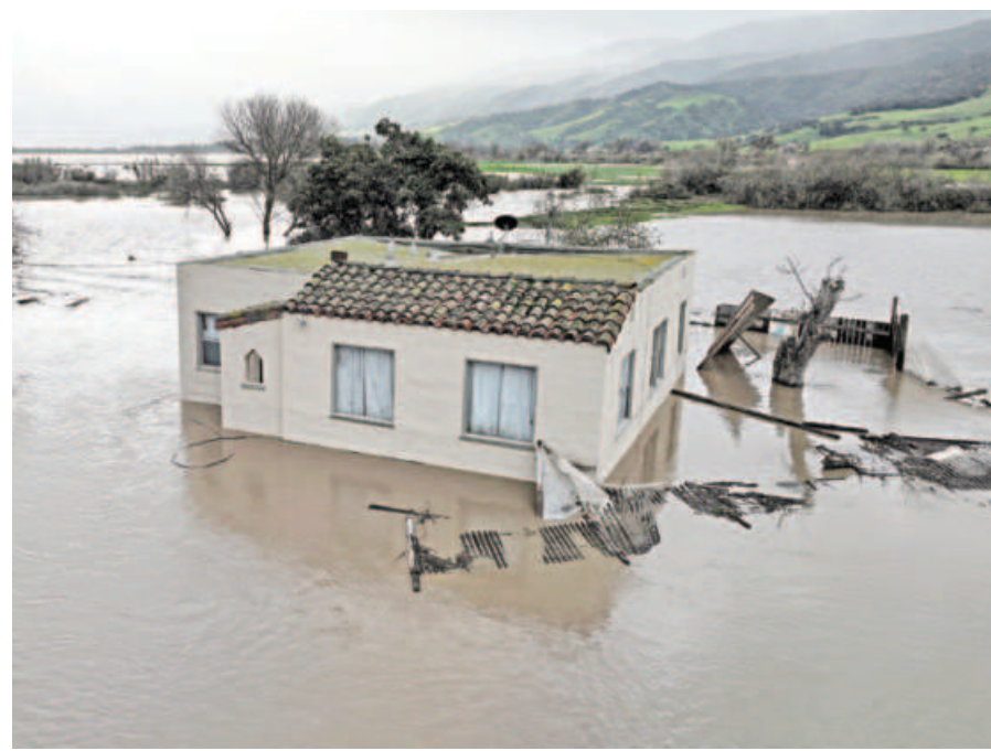
In an aerial view, a home is seen submerged in floodwater as the Salinas River begins to overflow its banks in Salinas, California, US, on Friday. The flood situation in California may worsen by the weekend, forecasters warned Friday. PHOTO: AFP
