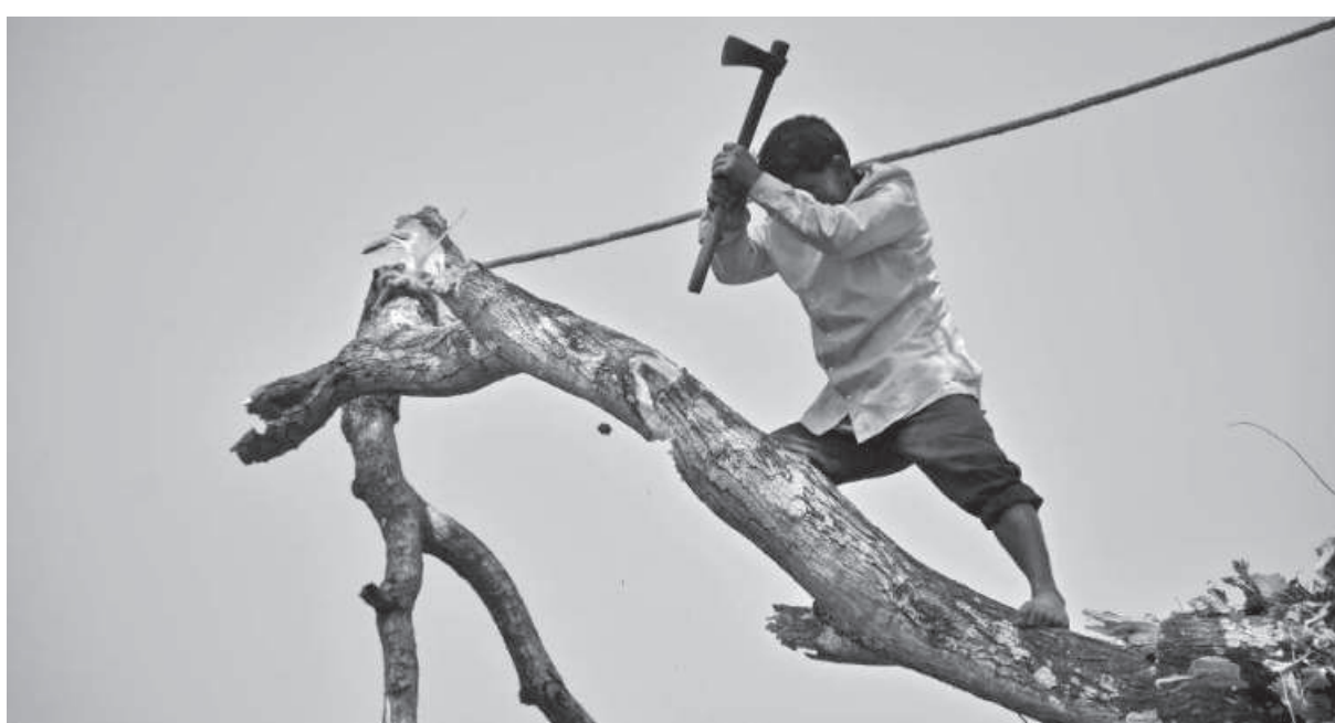
In order to widen Dhaka-Barishal highway, the authorities have decided to cut trees on the side of the road. Although there's a rope to ensure that the branch doesn't fall on the road and injure passers-by, there's no harness to save the man cutting the branch from a deadly fall. This photo was taken recently.
