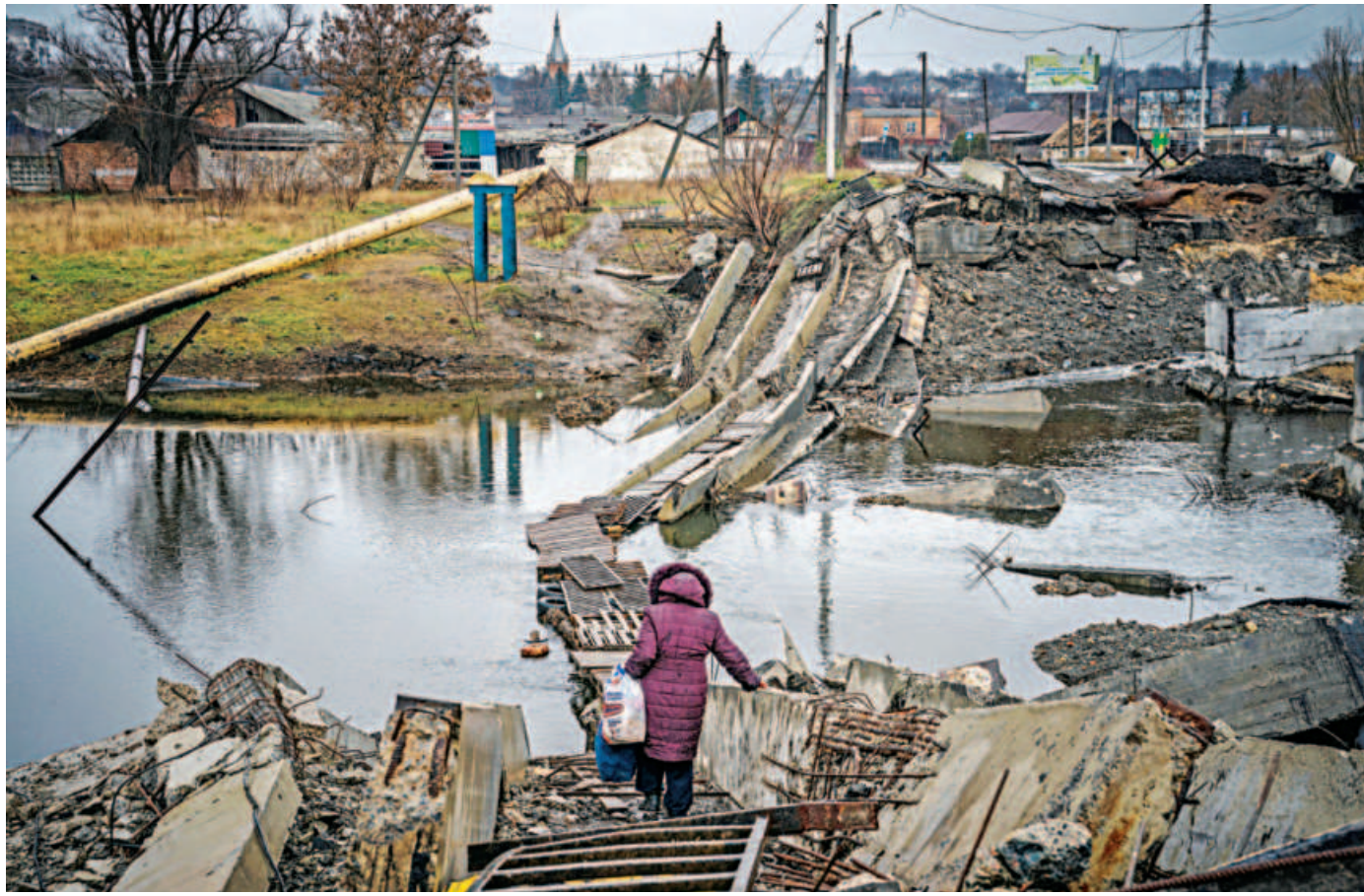
A woman crosses a destroyed bridge in Bakhmut, Donetsk region, yesterday. Russia and Ukraine have both suffered heavy casualties in the fight for Bakhmut, and most of the city's pre-war population of 70,000 have left for safer territory, leaving behind cratered roads and buildings reduced to rubble and twisted metal. PHOTO: AFP
