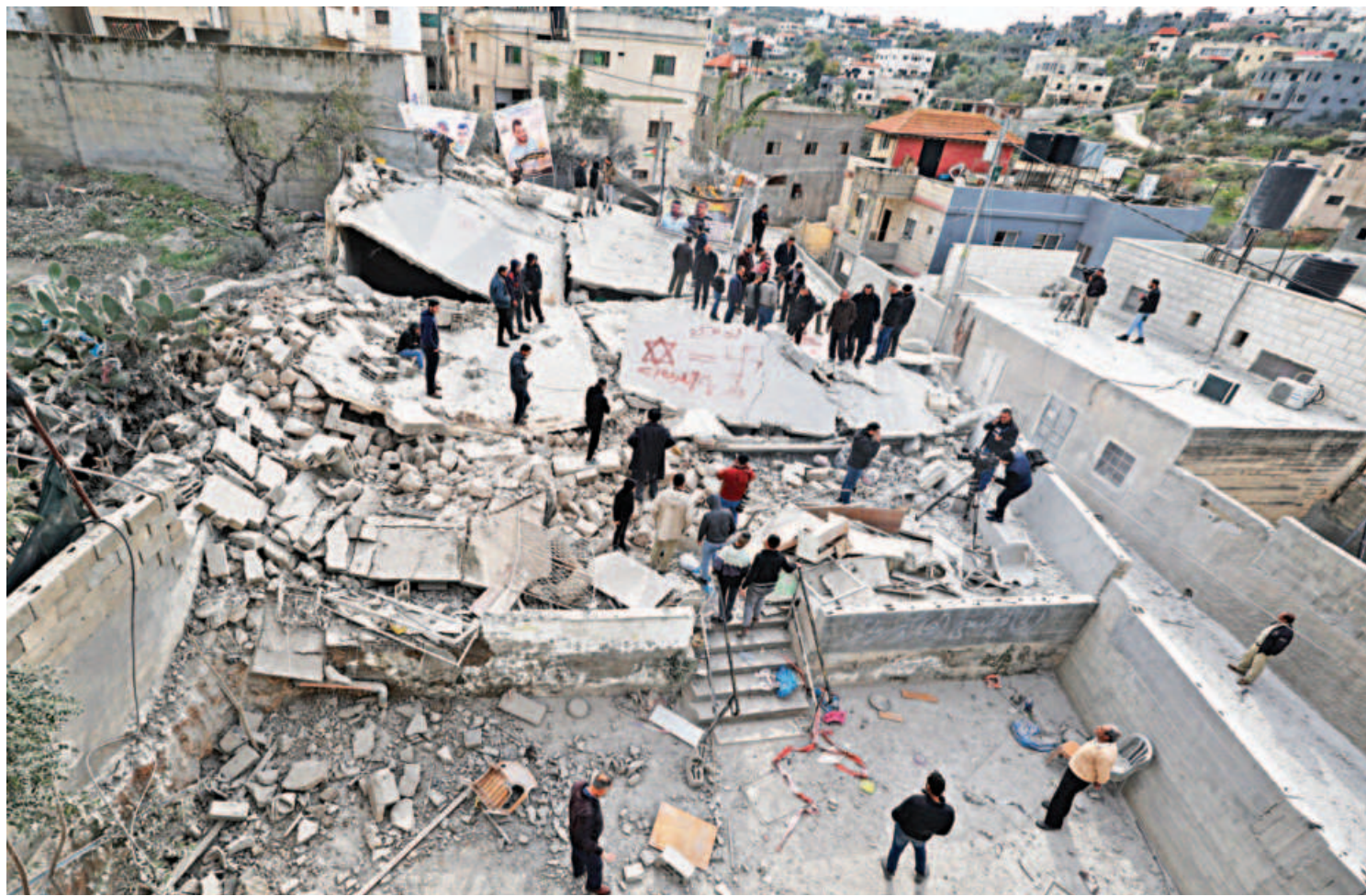
People inspect the rubble of a house that was demolished by Israeli soldiers, in the village of Kafr Dan in Jenin, in the occupied West Bank, yesterday. The Israeli army killed two Palestinians in a West Bank raid yesterday as it demolished the homes of two Palestinians accused of killing an Israeli soldier, Palestinian officials said.
