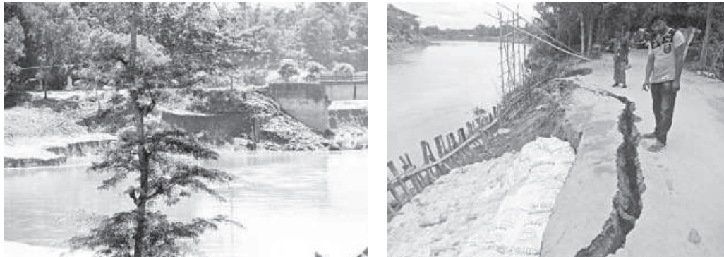
The river protection dam on the bank of Moulvibazar's Monu river remains unrepaired, as a project worth Tk 996.3 crore to protect three upazilas of the district from flooding is in limbo due to financial crisis. This photo was taken recently.
