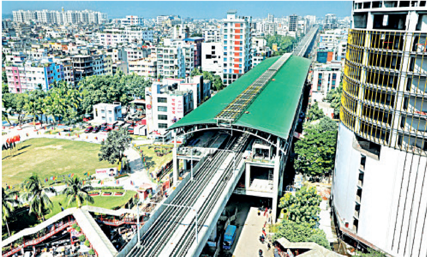
Construction work of the metro rail near the Mirpur-10 intersection. The photo was taken in January, 2022.
