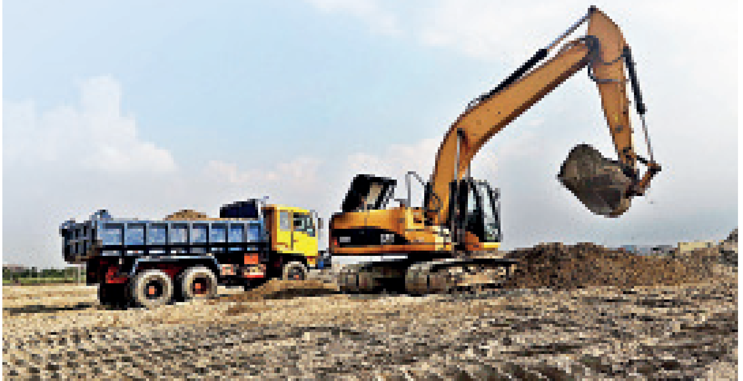
An excavator at a metro rail depot site at Dia Bari of Uttara where the construction work of the country's first metro rail service began on June 26, 2016.
