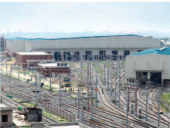
Trackworks and OCS at Uttara Depot
