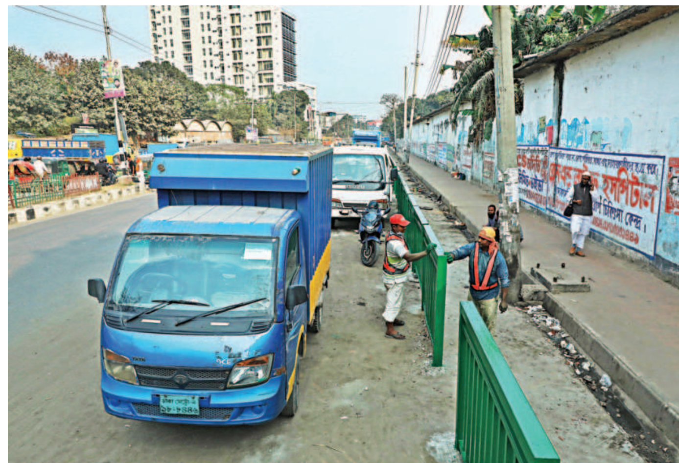
Dhaka North City Corporation has made a separate lane for Rickshaws by putting dividers on Tejaon Truck Stand Road.
