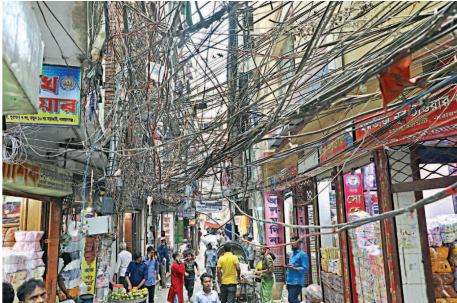
The ugly, tangled mess of overhead cables in Narayanganj's Nayamati area not only blemishes the skyline but also exposes pedestrians to great risks of accidents. The already concerning situation is exacerbated by the fact that this road is always full of people, as shops are situated on both sides. This photo was taken recently.
