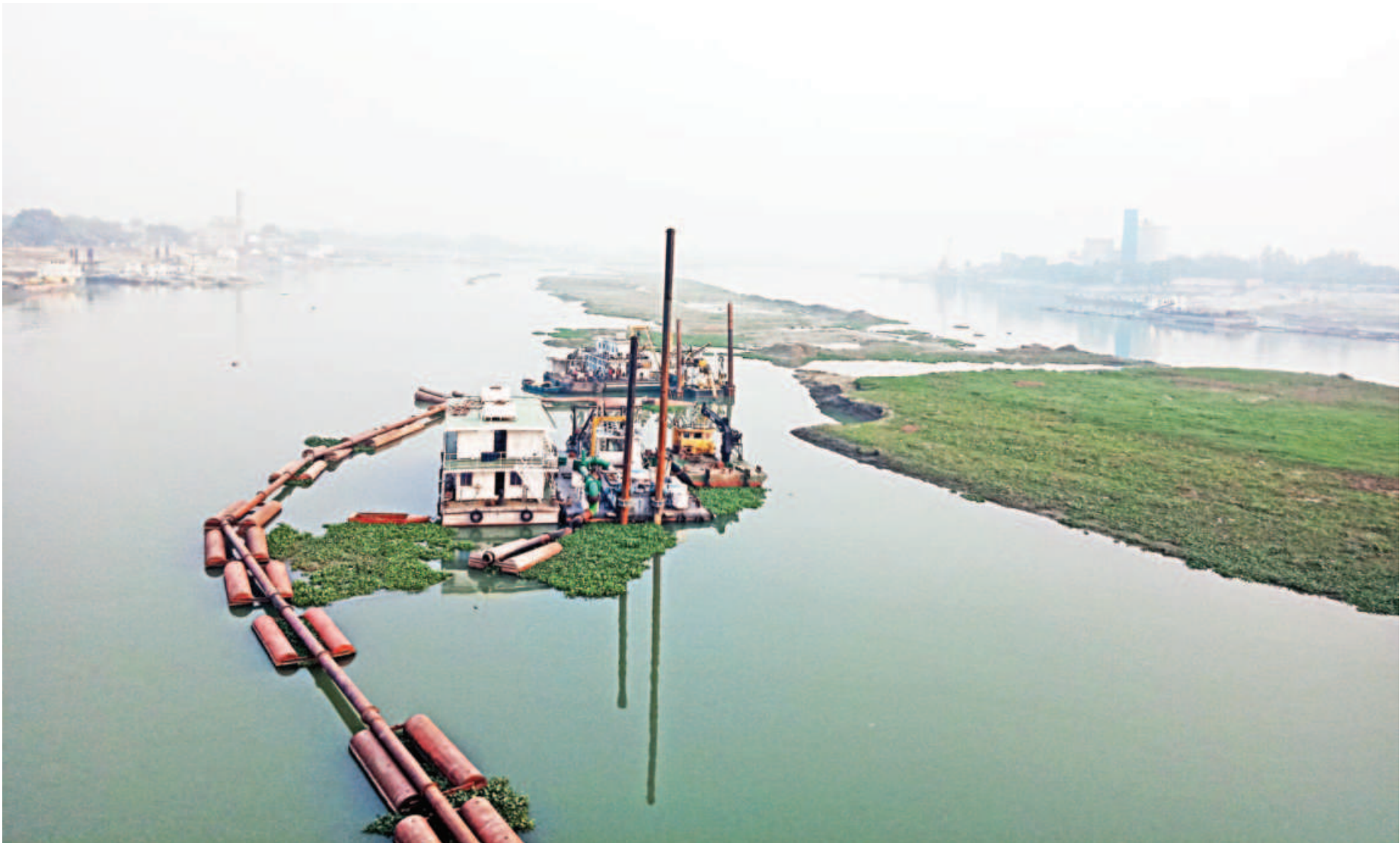
Dredging works are ongoing at Boral river in order to facilitate vessel movement centring the Baghabari river port. However, these seem more like stopgap measures as only widespread dredging across Jamuna river would help solve the navigability crisis that prevents large ships from docking at the port.
