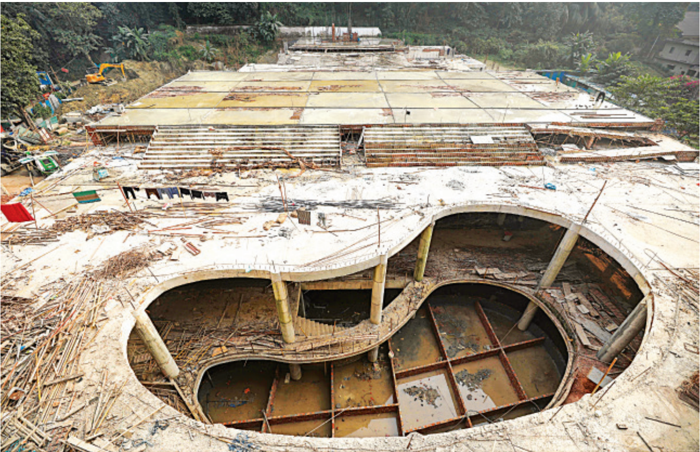
The construction of Shaheed Minar and Cultural Complex in Chattogram city's KC De Road area is yet to be completed. The Public Works Department started the work last year after knocking down the old one. The work was scheduled to be done before this Victory Day. For this, the city dwellers will have to celebrate the day at a Shaheed Minar temporarily built at the Municipal Model School and College. The photo was taken yesterday.
