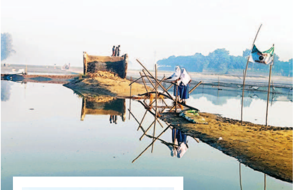
School students cross a bamboo bridge, with a half-built concrete one right in front. The incomplete bridge has been in this state for 27 years as the authorities concerned have taken no initiative to complete it. Locals have long been saying that their commutes would be made much easier if the bridge was functional.
