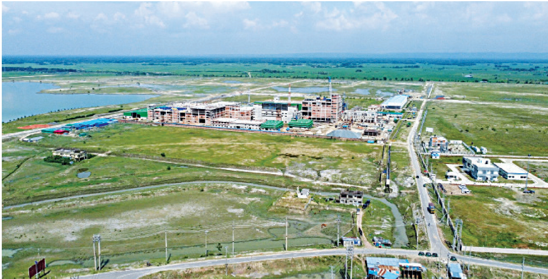
An aerial view of Bangabandhu Sheikh Mujib Shilpa Nagar in Mirsarai, Chattogram. Fenix Garment will set up a factory in Bepza Economic Zone of the Shilpa Nagar to produce high-end apparel products, including sports and motorcycle safety jackets, coveralls and hospital gowns.
