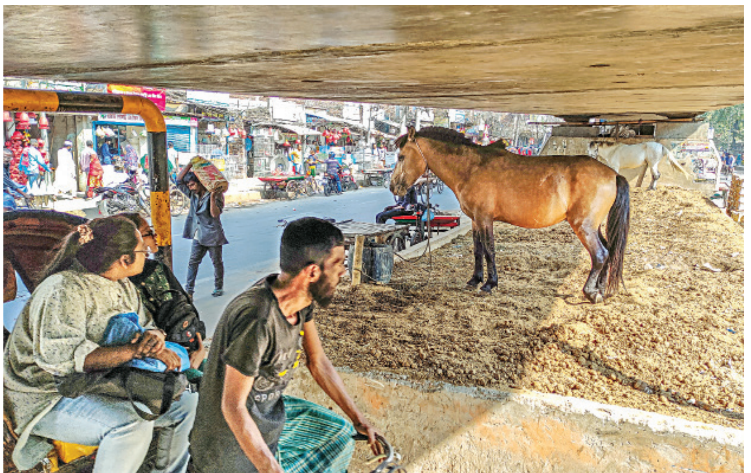
The empty spaces underneath Mayor Hanif Flyover seems to be up for grabs for anyone to use. Before, there used to be barricades preventing people from using this space. But now, horses are kept there and the local businessmen have turned the space into a makeshift stable. This photo was taken in Gulistan area yesterday.
