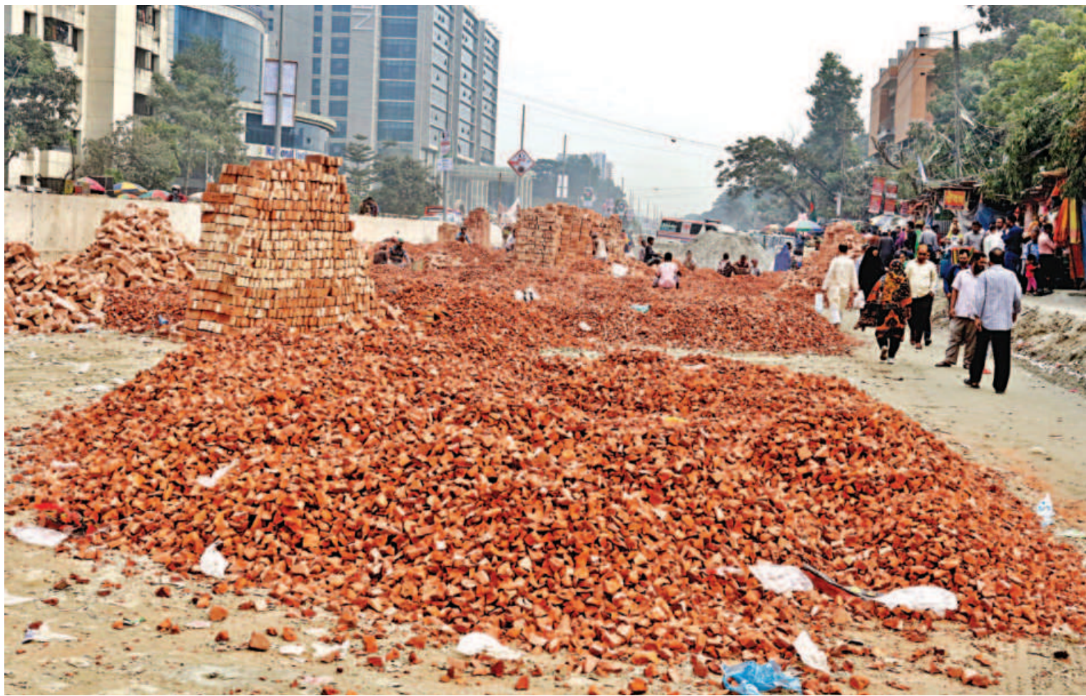
Brick chips are piled up on one side of the road beside Dhaka Shishu Hospital as development work goes on. As a result, vehicles pass from both directions on the other side of the road, resulting in traffic congestion, much to the dismay of patients and their attendees. This photo was taken recently.
