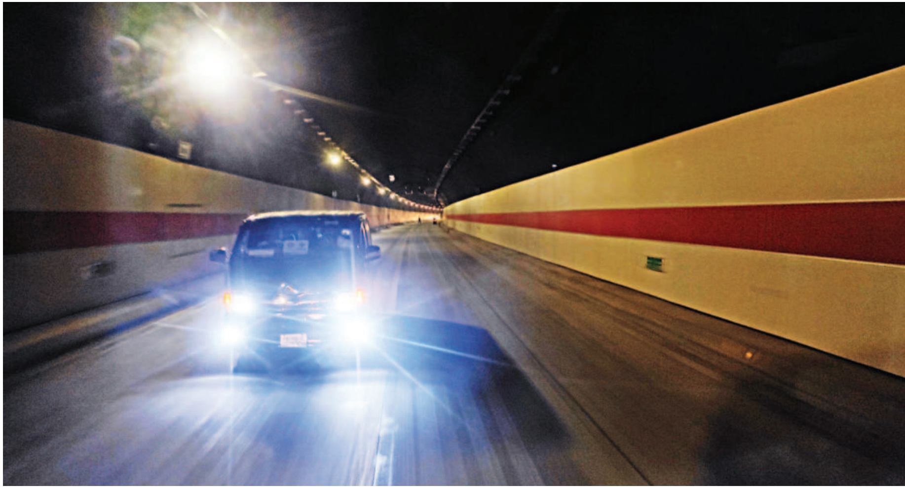
Bangabandhu Sheikh Mujibur Rahman Tunnel under the Karnaphuli river in Chattogram is expected to widen the scope for industrialisation and tourism in the country's south-eastern region. It is expected to be partially opened to traffic by the end of January next year. The photo was taken on Friday.
