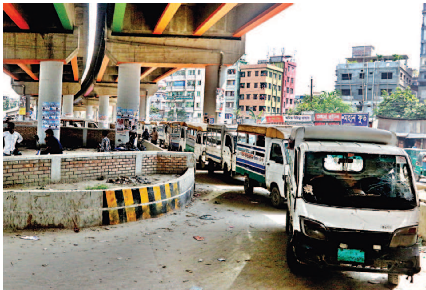
Illegally parked human hauliers leave almost no room for other vehicles under an overpass of Dhaka-Mawa expressway in the capital's Jurain. The photo was taken yesterday.
